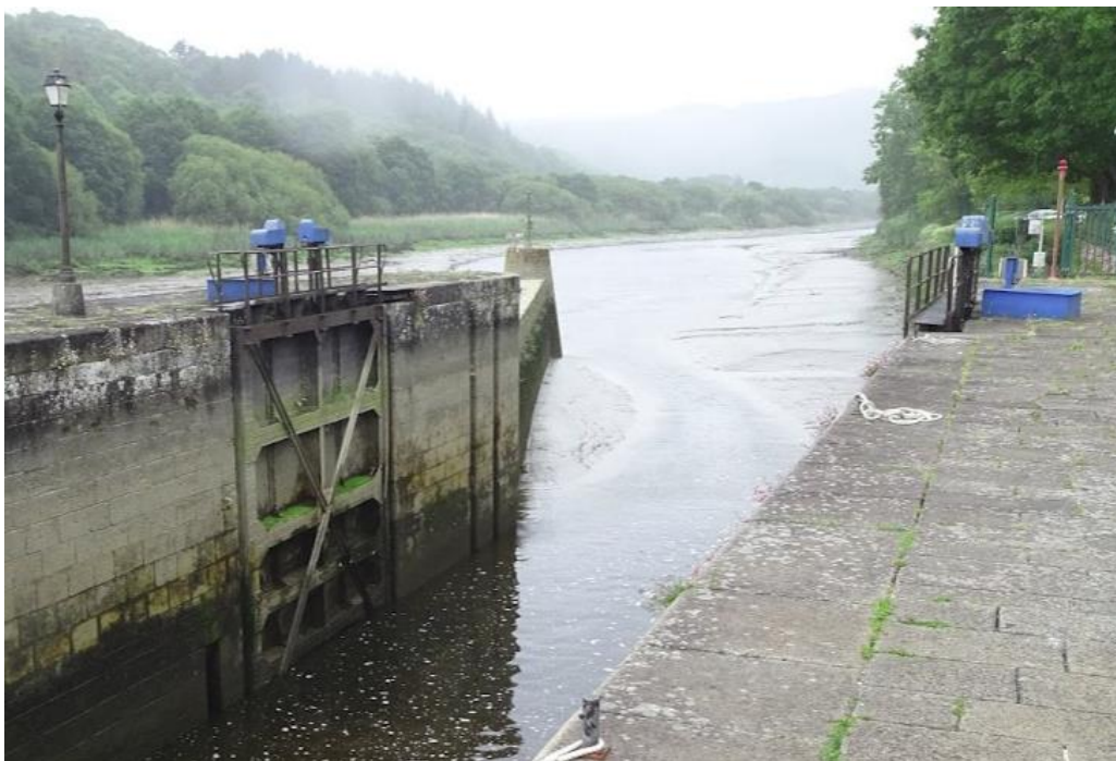
Gully Glaz lock – looking downstream
