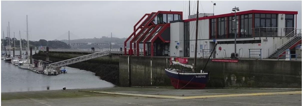
The Harbour office and facilities
