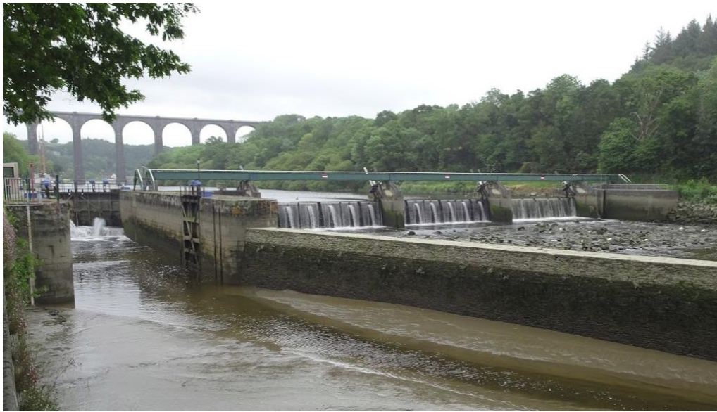
GUILY GLAZ lock looking upstream
