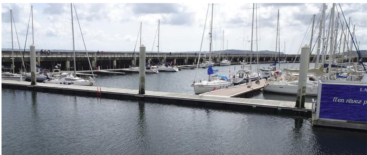
Chateau marina visitors pontoons on the left and middle. Some facilities on the pontoon
